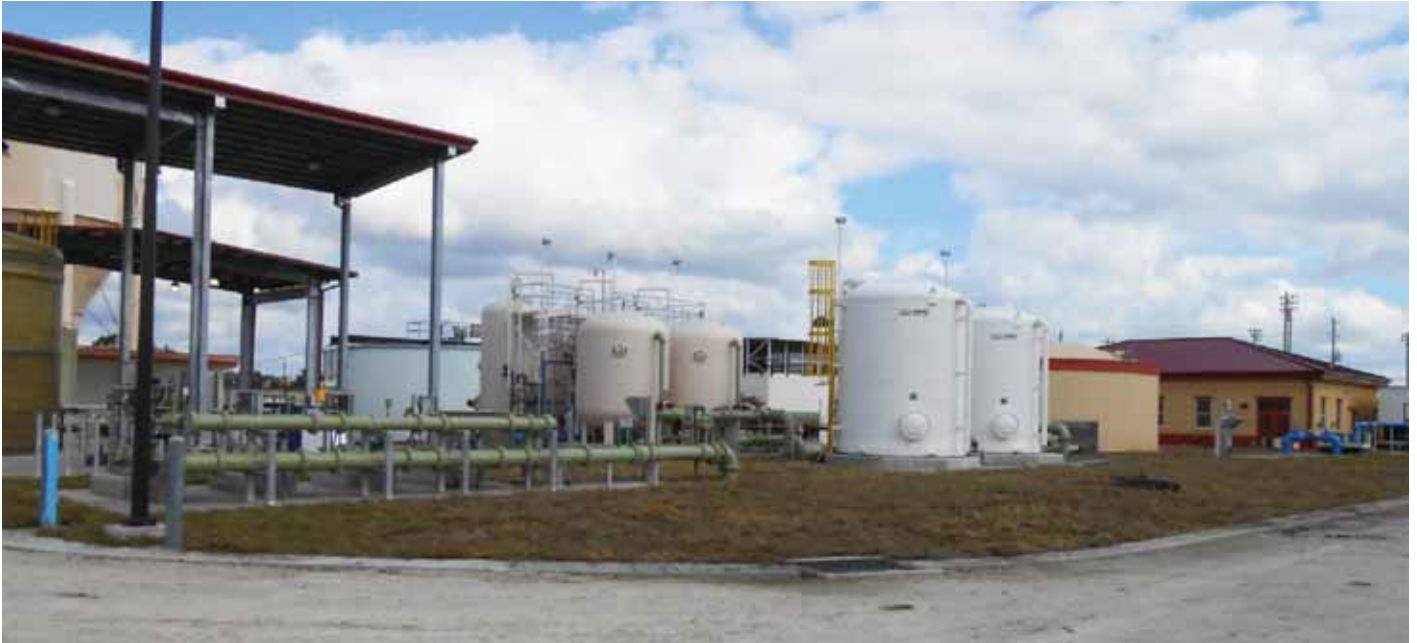
Figure 2. New Arcadia Ion Exchange Water Treatment Plant
